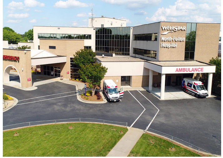
Wellstar North Fulton Hospital
