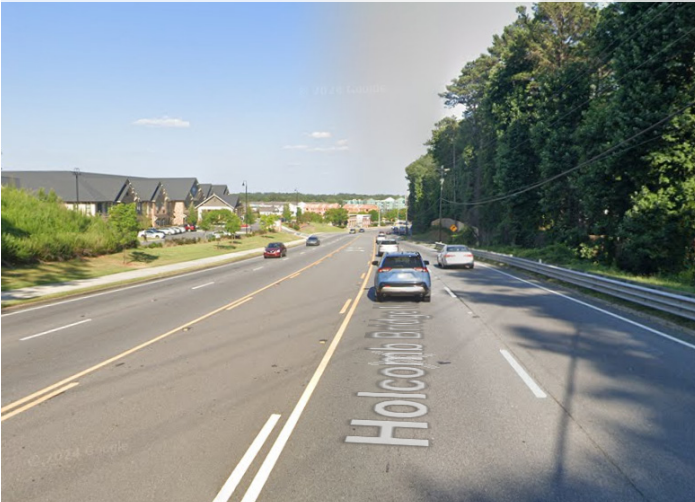
Holcomb Bridge Road
