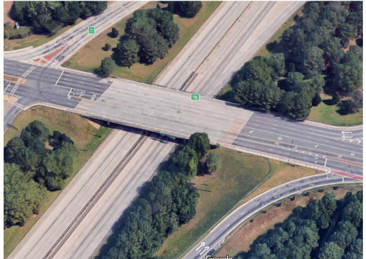
Holcomb Bridge Road/GA 400
